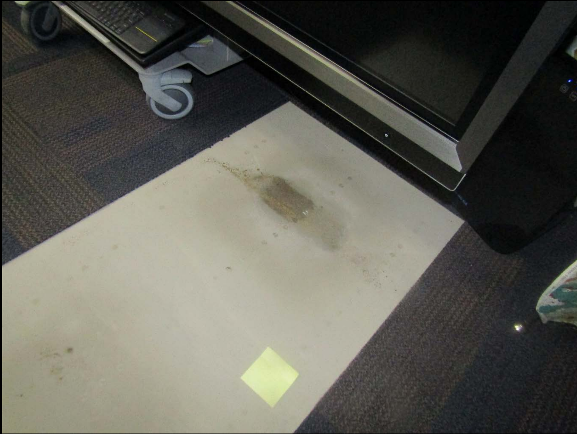
Photo 7. Example of Floor Staining and Liquid Water Under Carpet, Room D2
