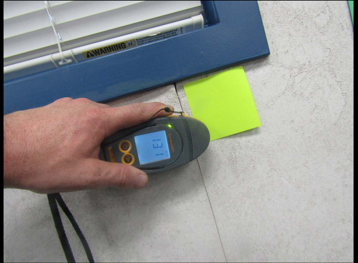
Photo 8. Example of Moisture Meter Measurement Near Peeling Wall Paper, Room E4
