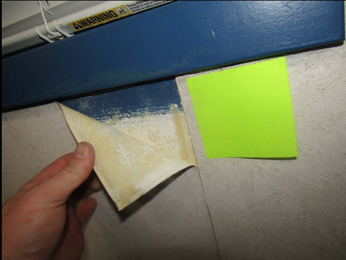
Photo 9. Example of Inspection of Wallpaper Backing and Gypsum Drywall, Room E4
