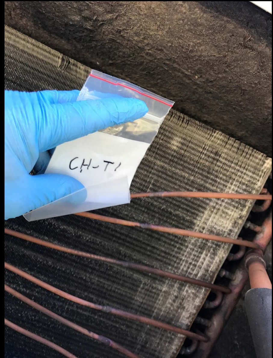
Photo 2. Surface Sample from AHU on Room 33
