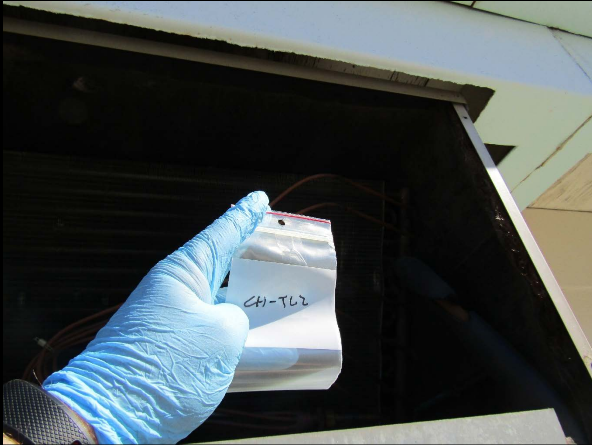
Photo 3. Surface Sample from AHU on Room 37
