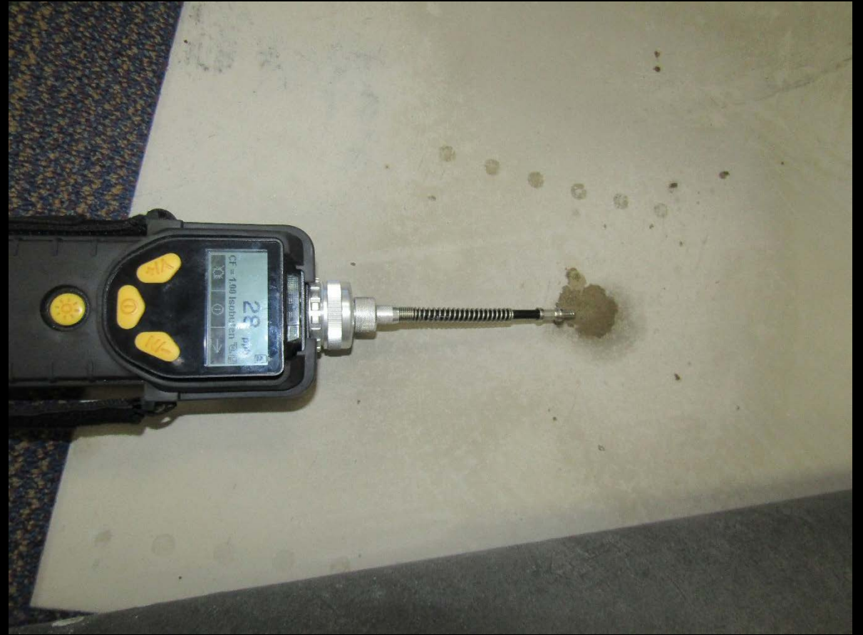
Photo 4. Example of Floor Staining and Liquid Water Under Carpet, Room E2
