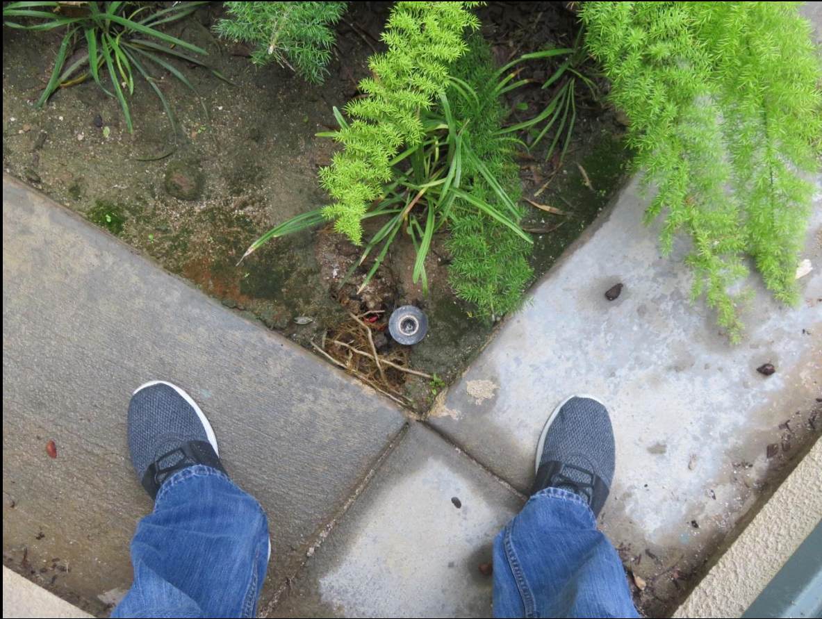
Photo 5. Atrium, Possible Broken irrigation Line, North Park Elementary
