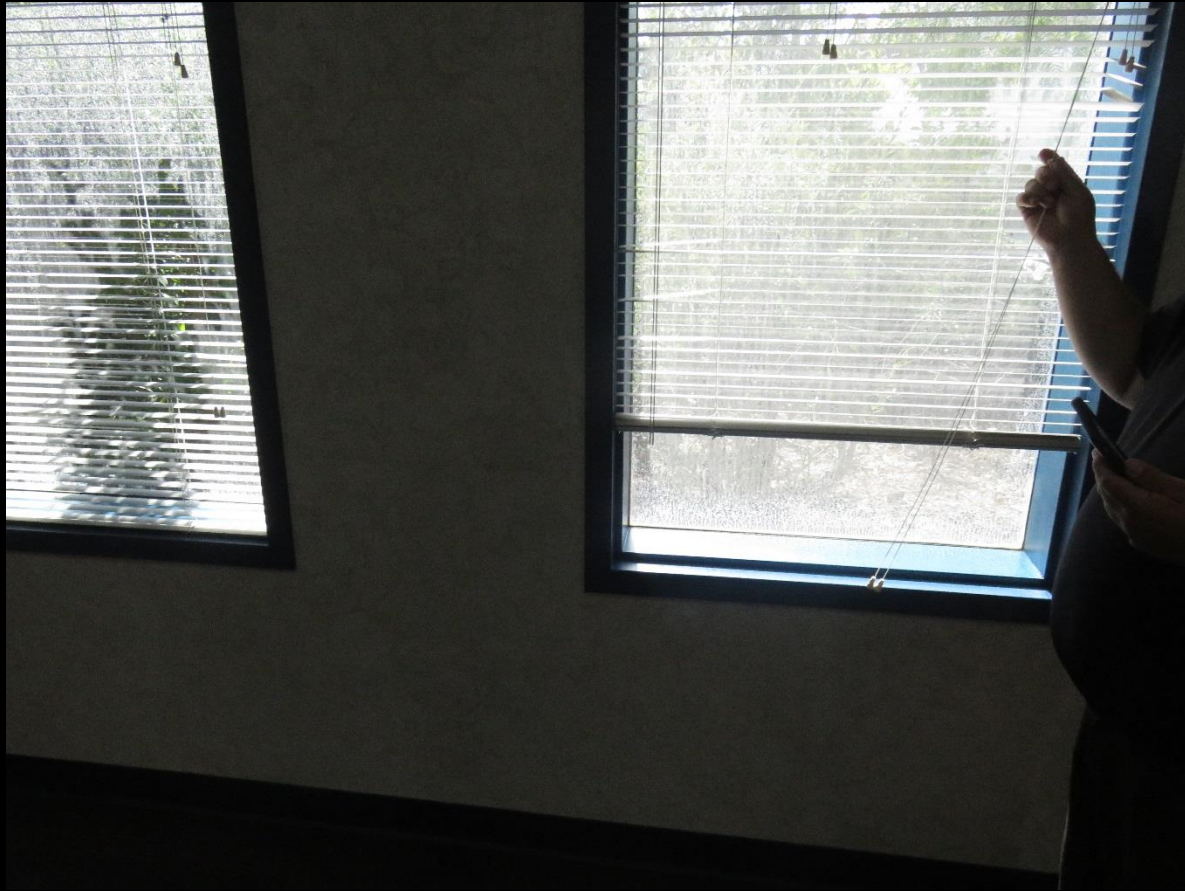
Photo 11. Hard Water Staining on Window, Bridgeport Elementary
