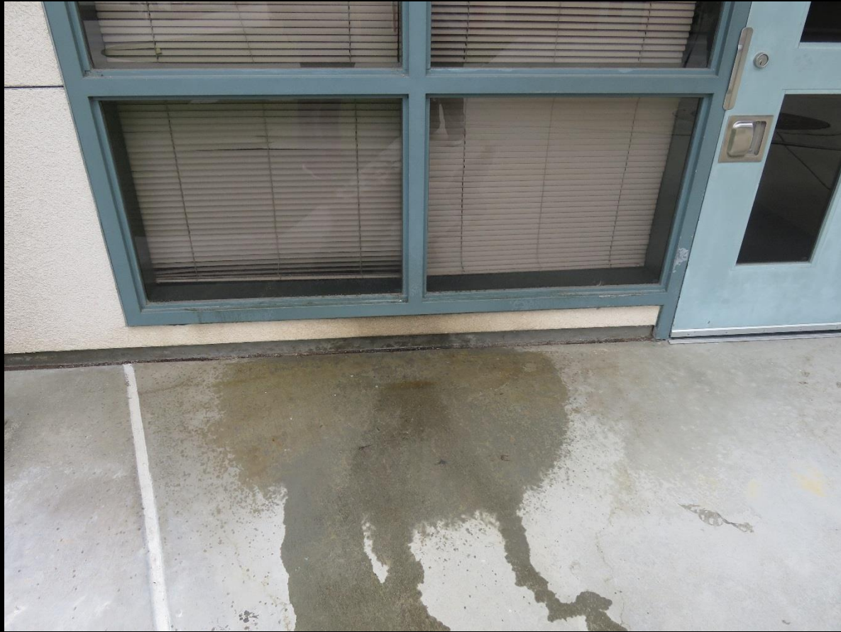
Photo 7. Stain on Ground below Downspout, North Park Elementary
