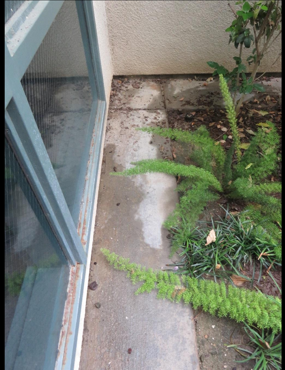
Photo 4. Atrium, Staining on Concrete, North Park Elementary
