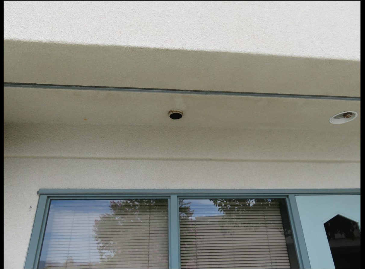
Photo 6. Representative Downspout Outside of Classroom, North Park Elementary
