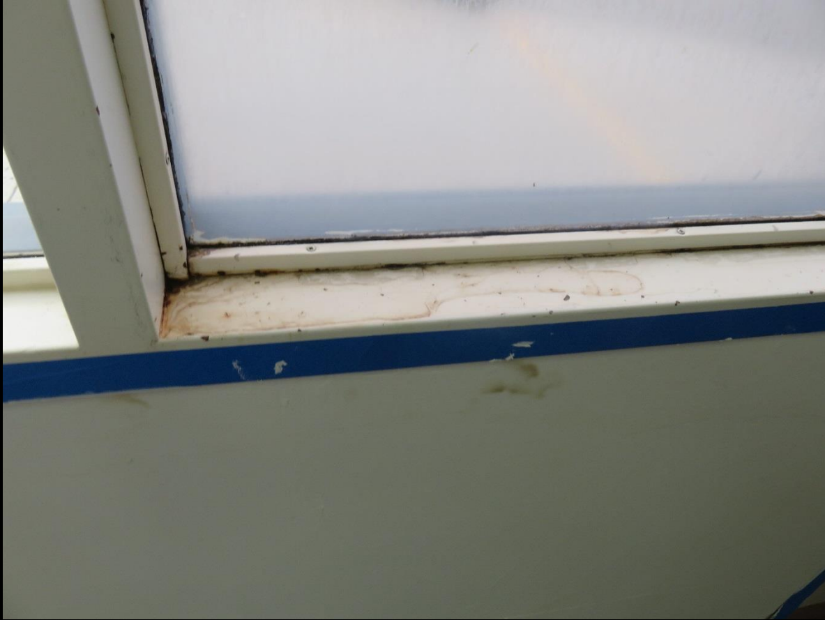
Photo 9. Staining on Window Sill at Remediation Location, Mountain View Elementary
