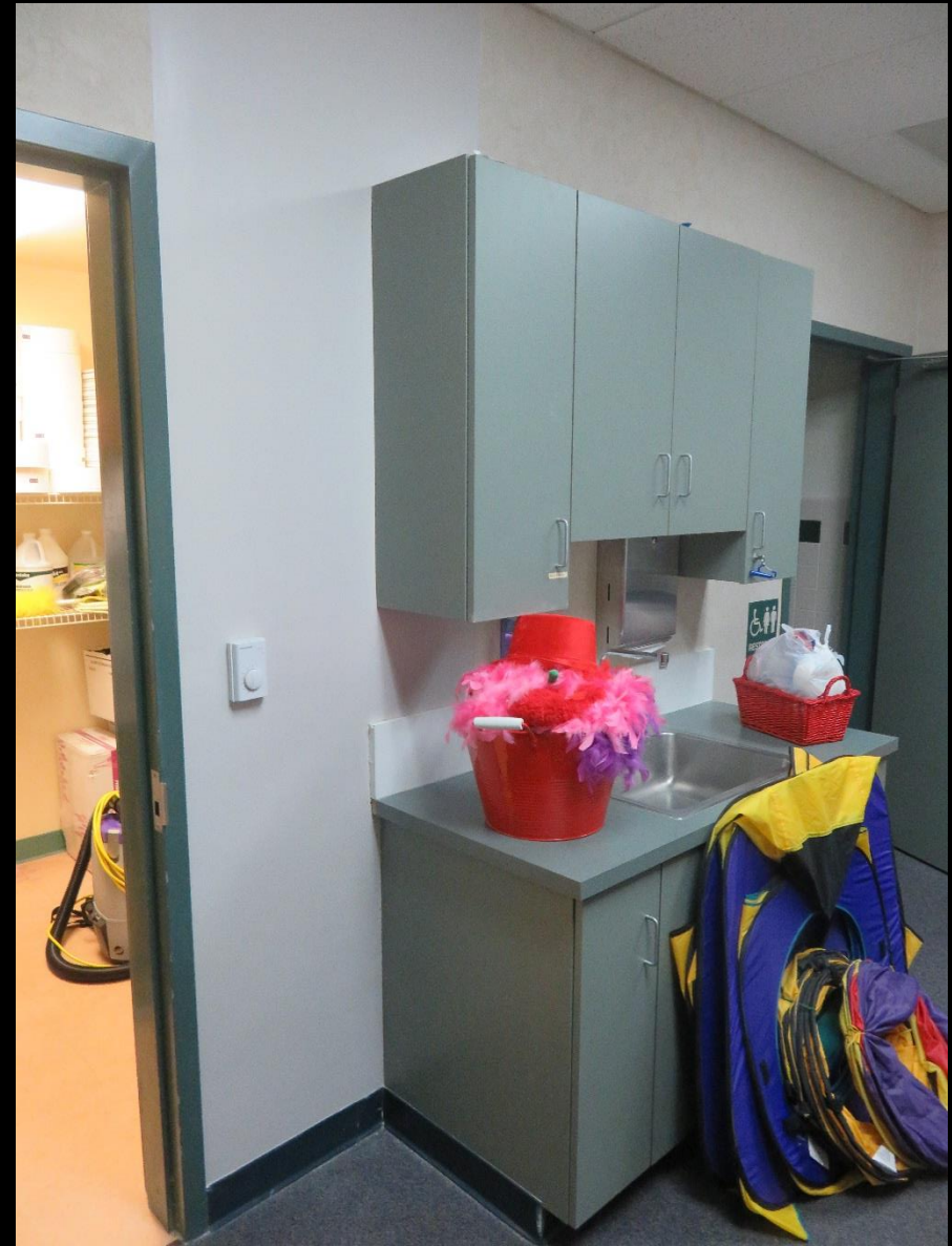
Photo 2. Remediated Area, Classrooms 1 and 2, North Park Elementary
