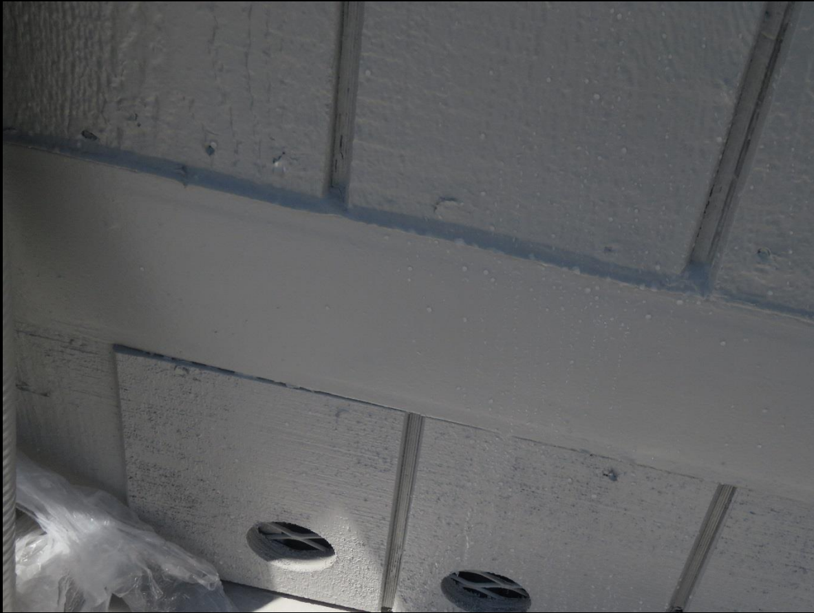
Photo 1. Condensate Line Dripping on Siding, Unit 39A, Emblem Elementary
