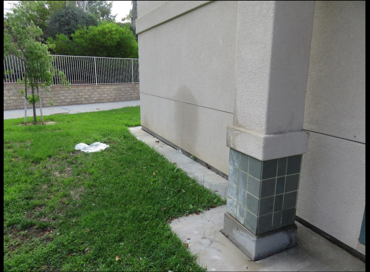
Photo 8. Possible Irrigation Water Stain on Building Exterior, North Park Elementary
