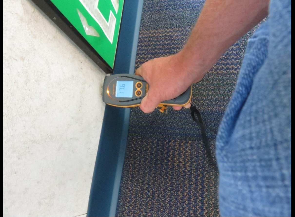
Photo 10. Wet Drywall Near Exit Sign, Classroom C1, Bridgeport Elementary
