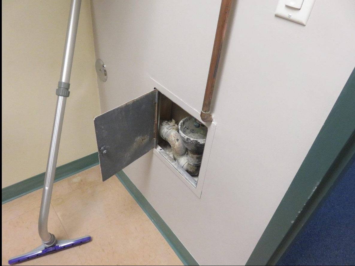
Photo 3. Remediated Area, Classrooms 1 and 2, North Park Elementary
