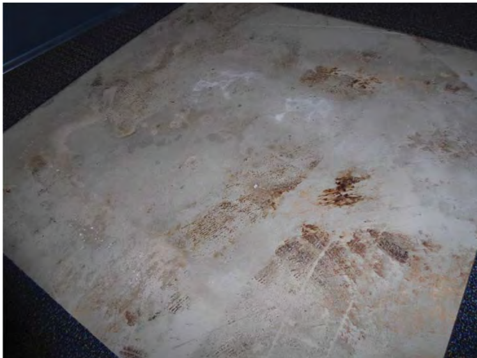
Mositure Dome Prep, A31 - JS 6-3-17 (12)
