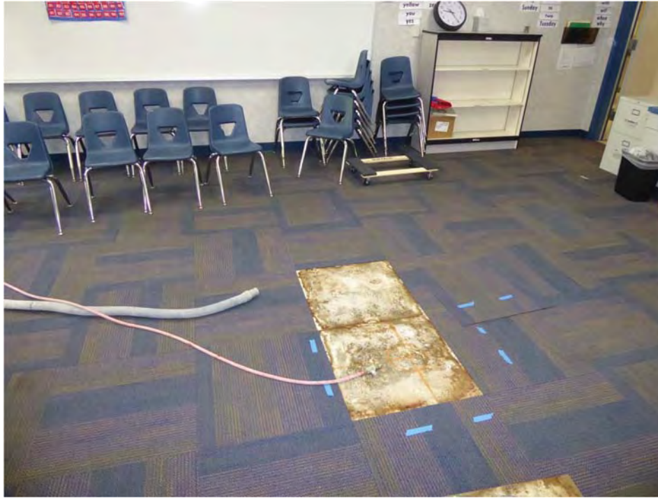
Mositure Dome Prep, A11 - JS 6-3-17 (9)
