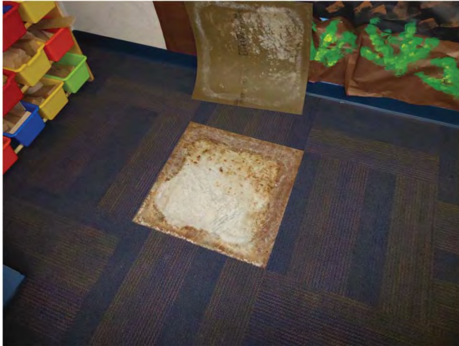
Mositure Dome Prep, A11 - JS 6-3-17 (7)
