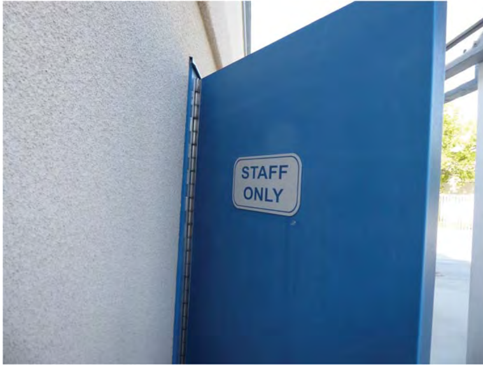
Mositure Dome Prep, A31 - JS 6-3-17 (3)
