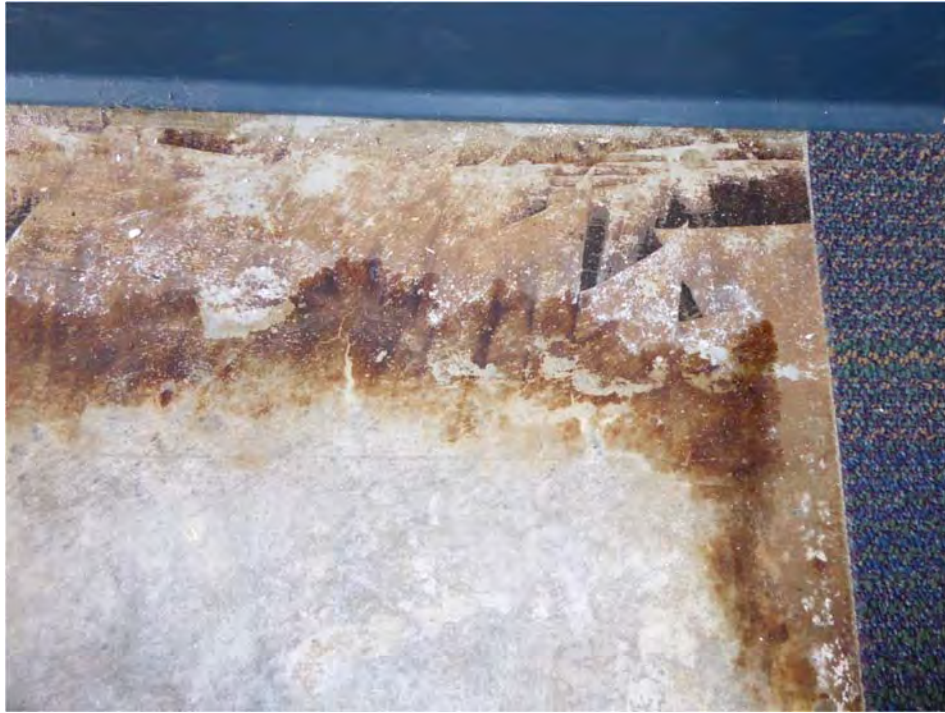
Mositure Dome Prep, A11 - JS 6-3-17 (5)
