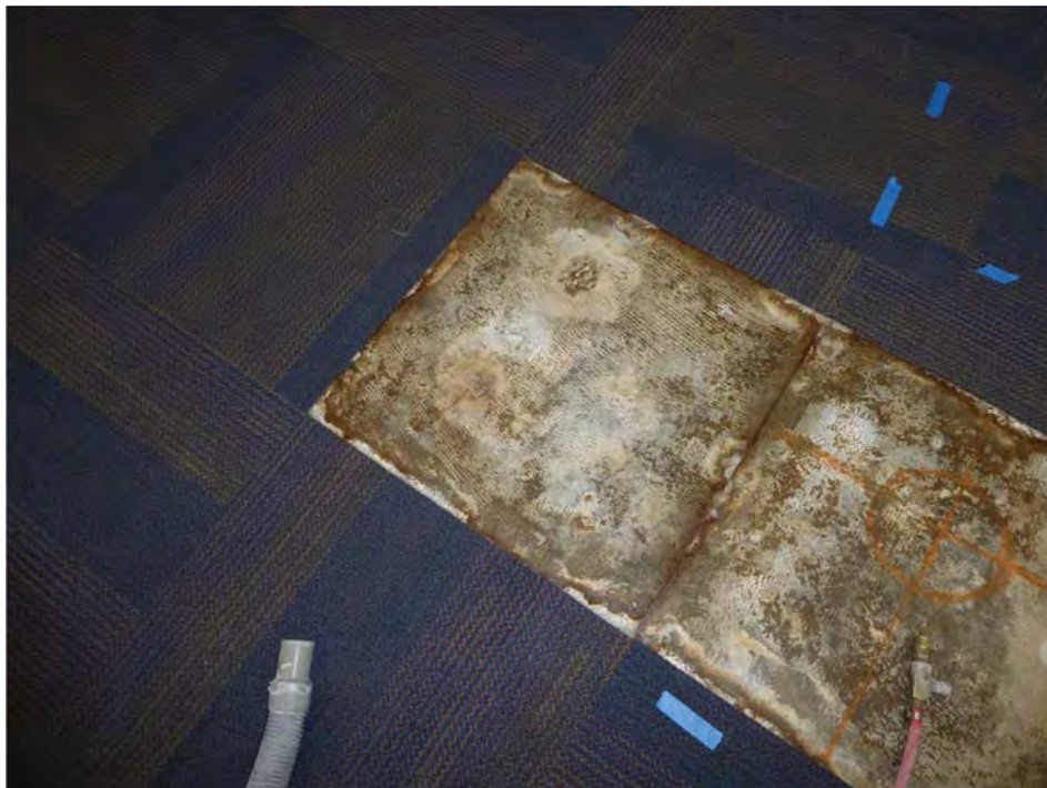
Mositure Dome Prep, A11 - JS 6-3-17 (10)
