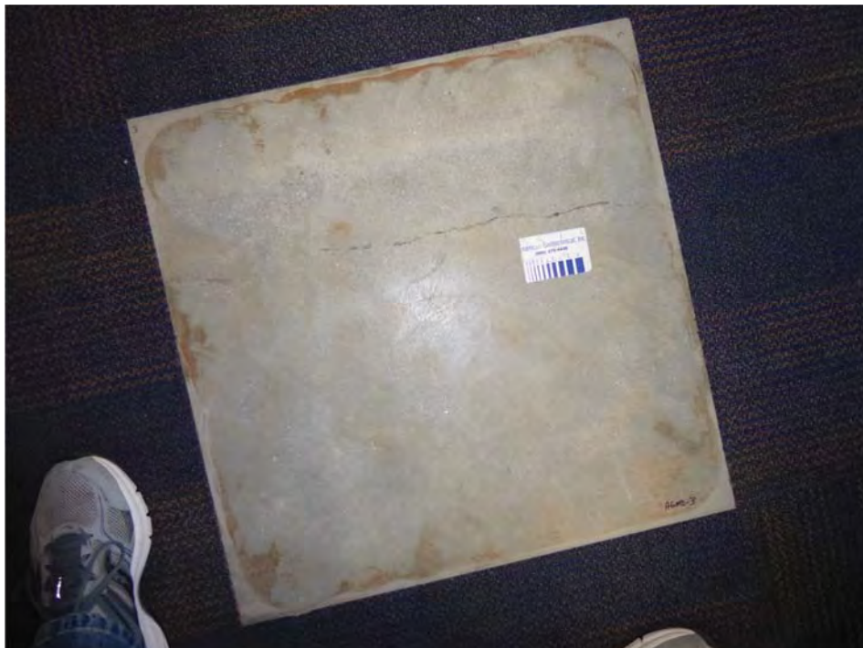
Mositure Dome Prep, A31 - JS 6-3-17 (16)
