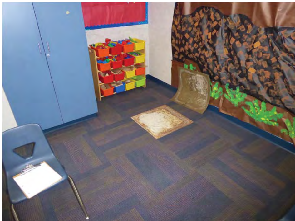
Mositure Dome Prep, A11 - JS 6-3-17 (6)
