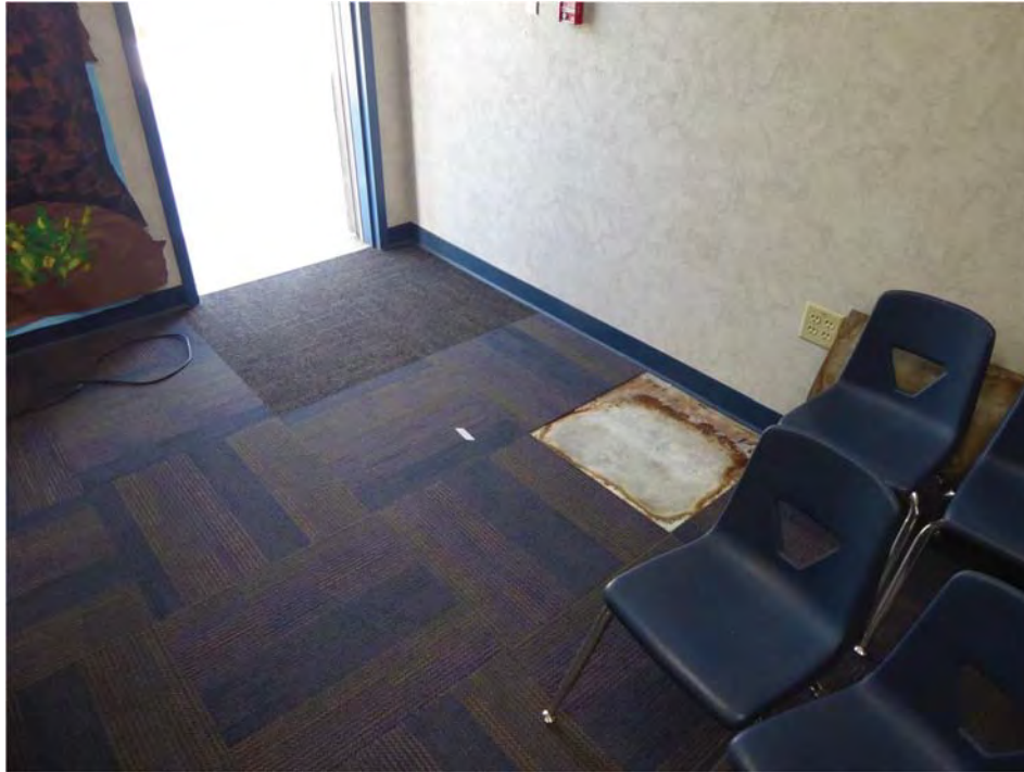
Mositure Dome Prep, A11 - JS 6-3-17 (3)
