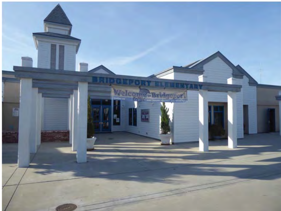
Mositure Dome Prep, A31 - JS 6-3-17 (2)
