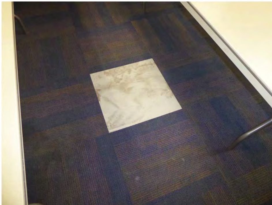
Mositure Dome Prep, A31 - JS 6-3-17 (14)
