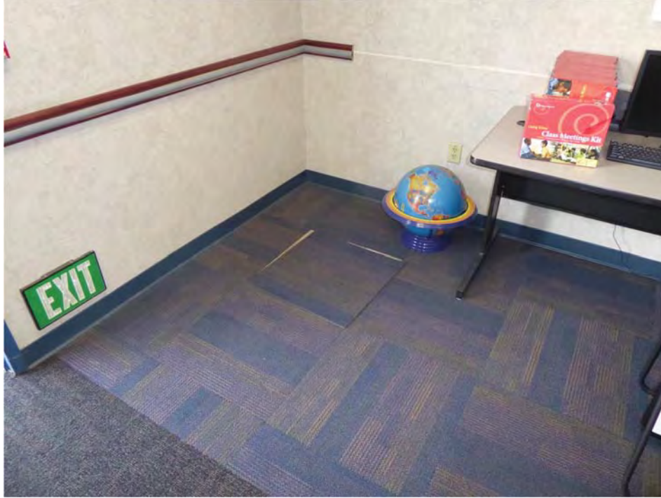
Mositure Dome Prep, A31 - JS 6-3-17 (5)
