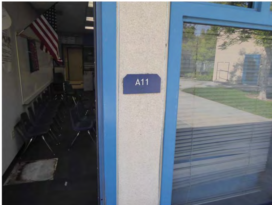
Mositure Dome Prep, A11 - JS 6-3-17 (2)
