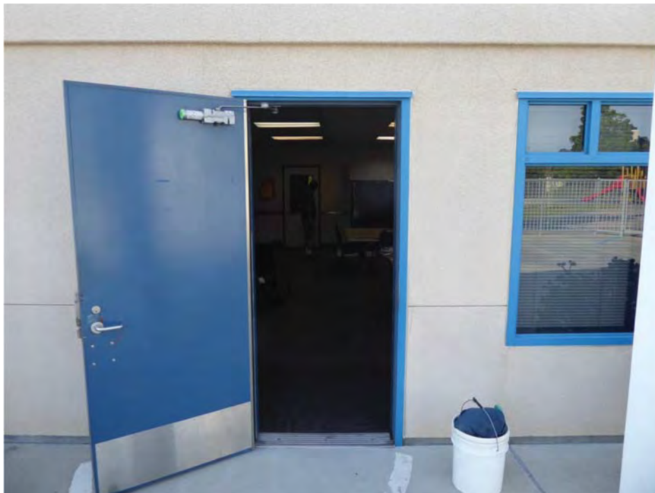
Mositure Dome Prep, A31 - JS 6-3-17 (4)
