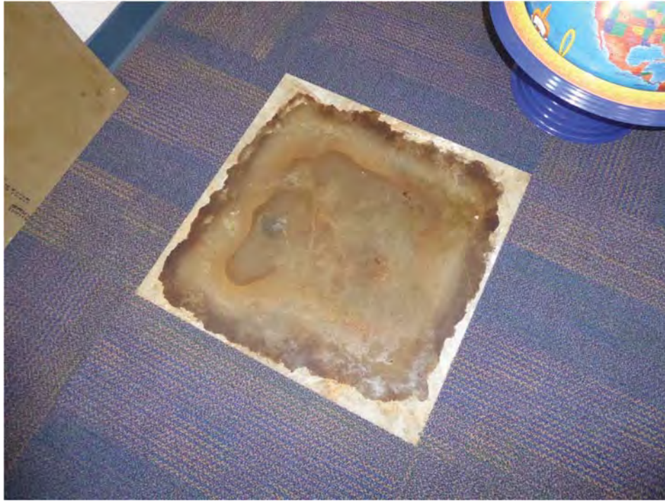
Mositure Dome Prep, A31 - JS 6-3-17 (7)
