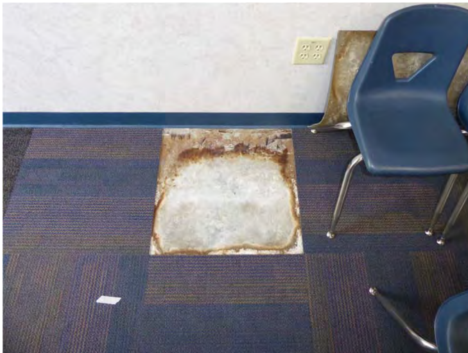
Mositure Dome Prep, A11 - JS 6-3-17 (4)
