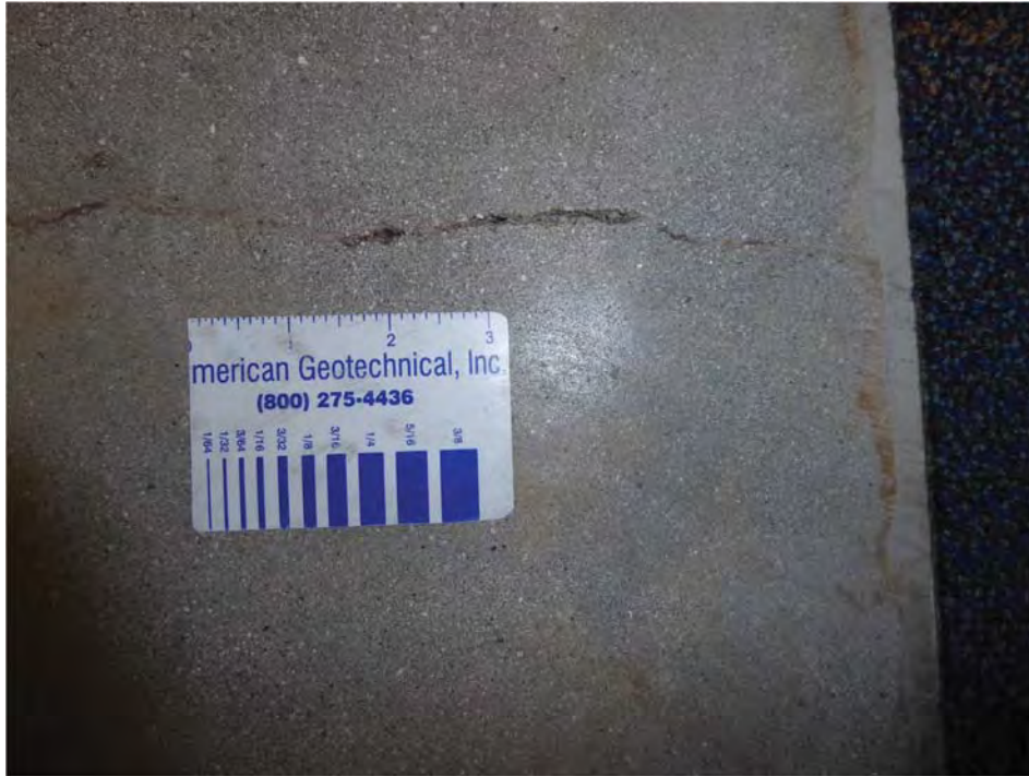
Mositure Dome Prep, A31 - JS 6-3-17 (17)
