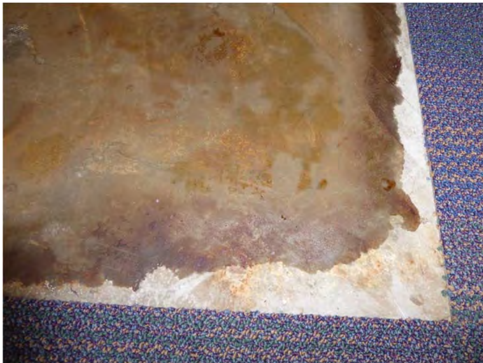
Mositure Dome Prep, A31 - JS 6-3-17 (8)
